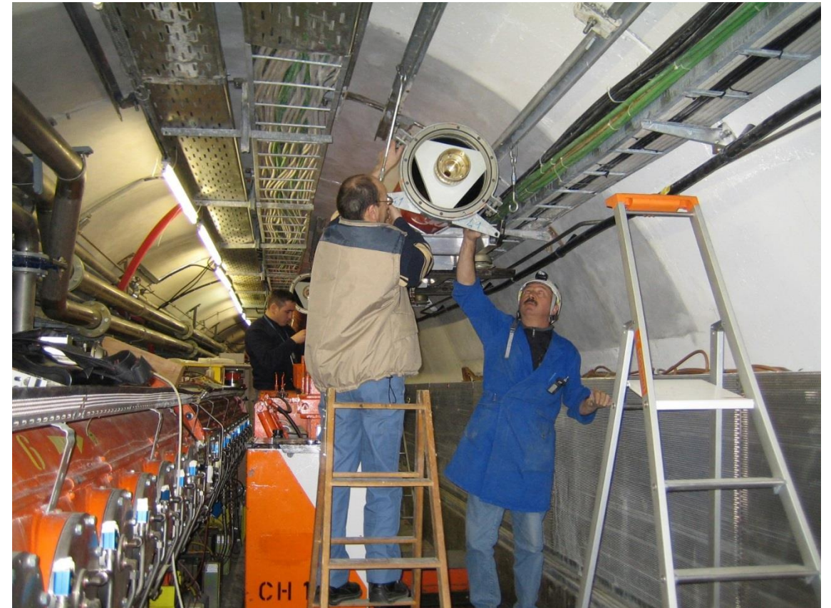
CERN SPS 200 MHz, 4 * 150 meters of 345 mm coaxial lines from the surface building to the cavities
