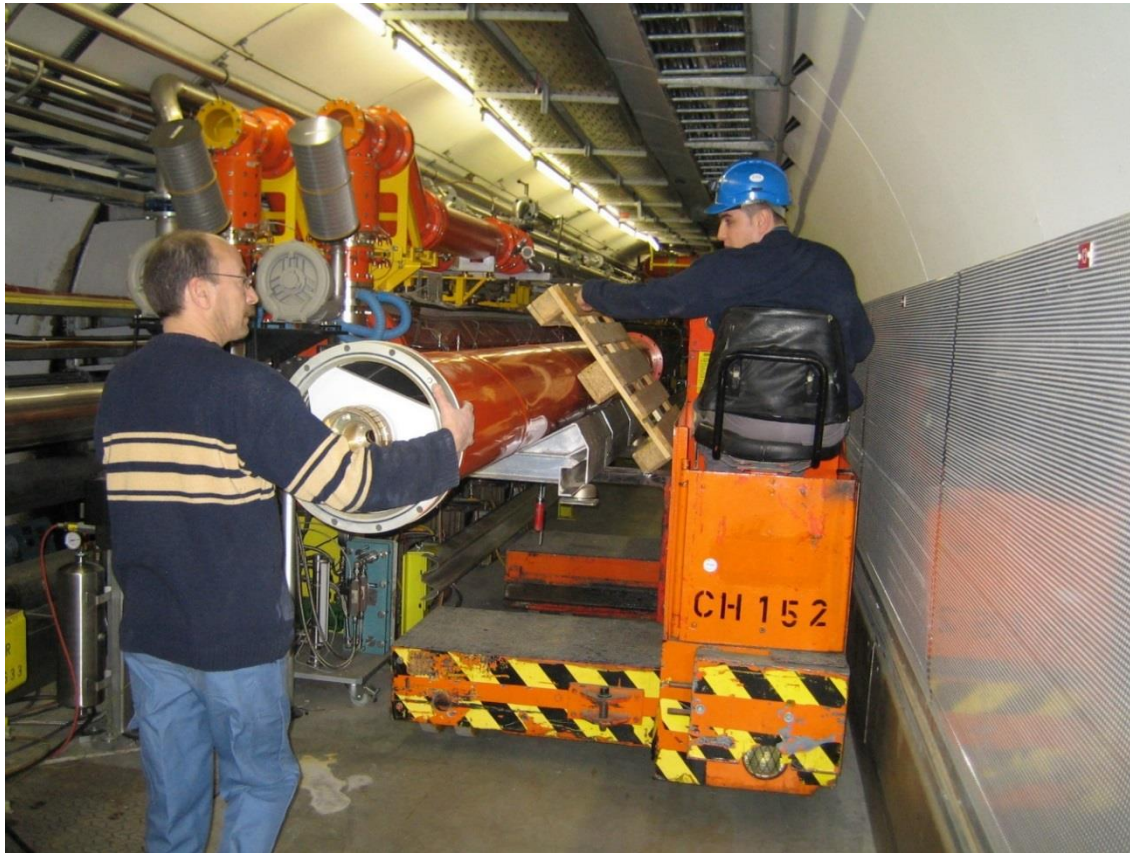
CERN SPS 200 MHz, 4 * 150 meters of 345 mm coaxial lines from the surface building to the cavities
